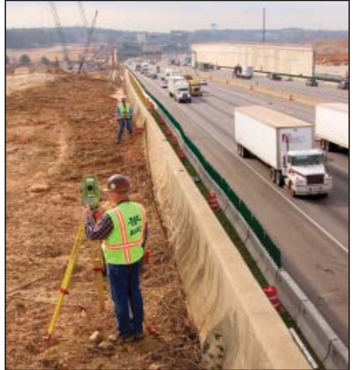
Surveyors verify control before constructing a new bent wall.
