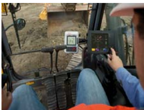
Leica Digger 3D being used by an operator on site.
